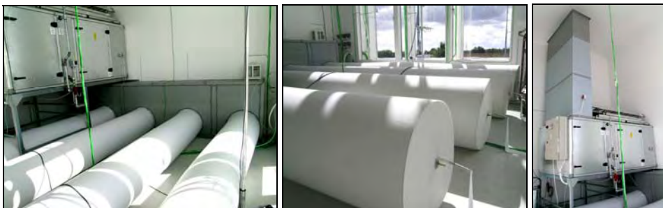
Figure 4. KE-low impulse fabric ducts in the experiment room (left, centre), Ventilation system in the experiment room (right).
