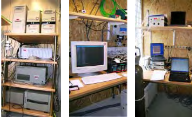
Figure 5. Equipment in the instrument room.
