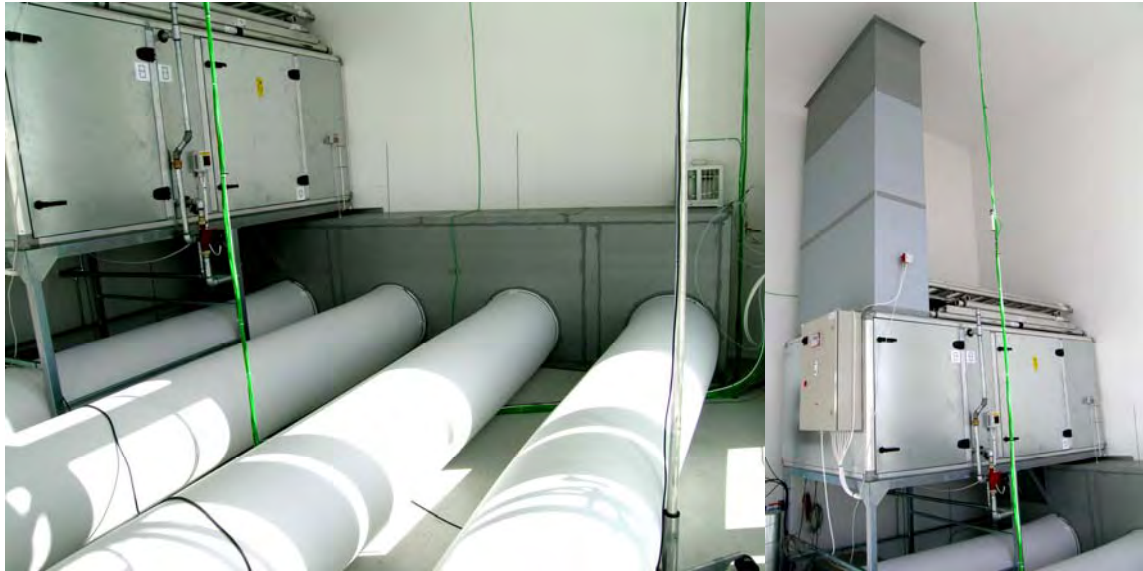
Figure 17. Ventilation recirculation system.
